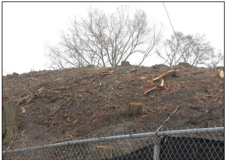
AFTER woodland clearing.
